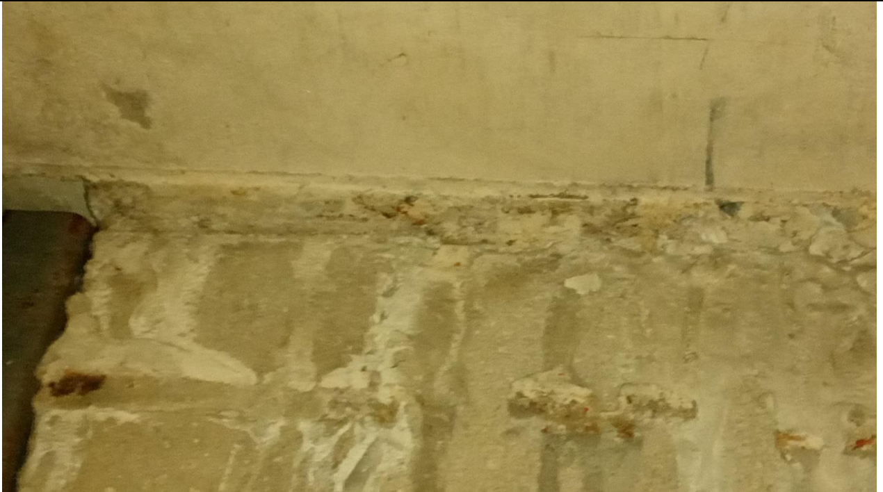
Photograph 9. (Location 1 in the central corridor area), shows the interface with a concrete column.
