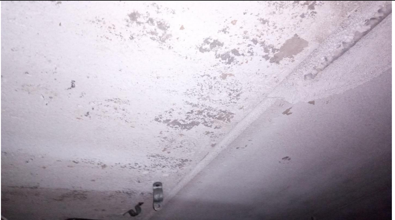
Photograph 3. (Location 1 in the Autoclave room), shows the soffit of the roof planks and some redundant pipe supports.
