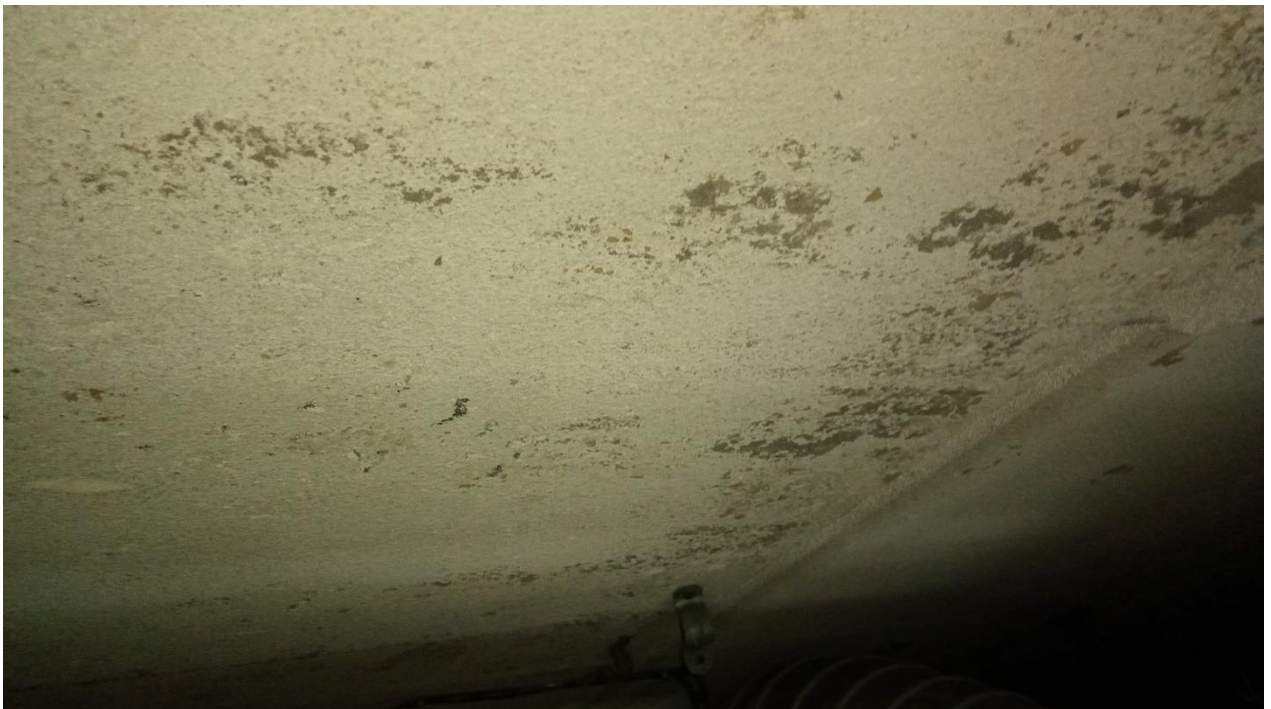
Photograph 4. (Location 1 in the Autoclave room), shows the soffit of the roof planks and some redundant pipe supports can also be seen screwed to the planks.
