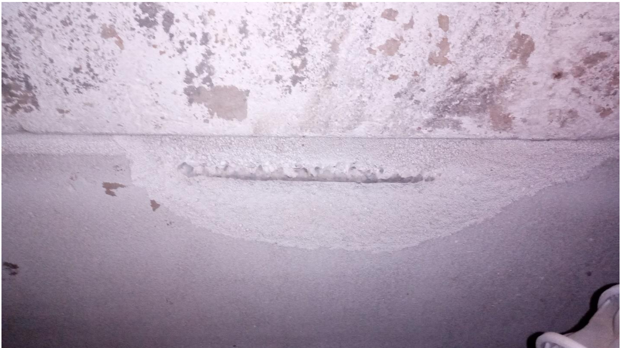
Photograph 2. (Location 1 in the Autoclave room), shows a spalled section of roof plank. Debris from the spalling could not be seen on the ceiling tiles. The aerated core of the lightweight concrete plank can be clearly seen to the damaged area, confirming that the planks are reinforced autoclaved aerated concrete (RAAC).
