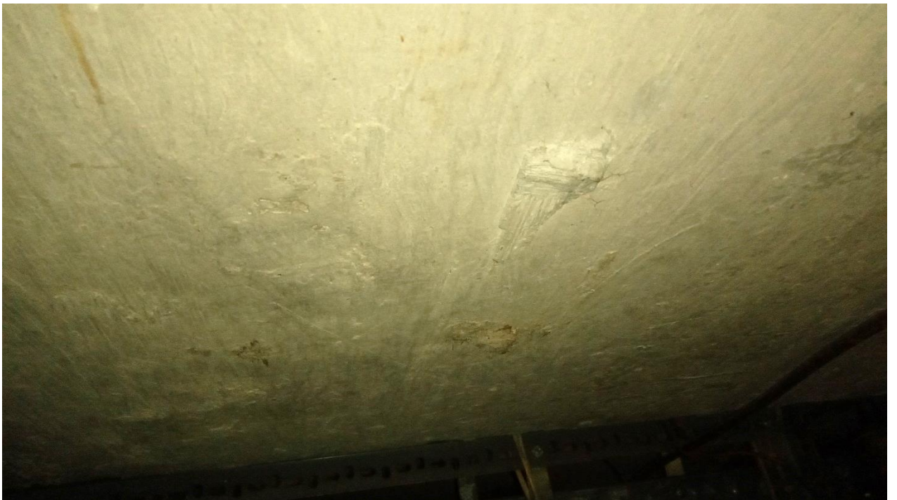
Photograph 6. (Location 1 in the central corridor area), shows the rough surface of the soffit of some roof planks. Some brown staining possibly from corroding reinforcement can be seen.
