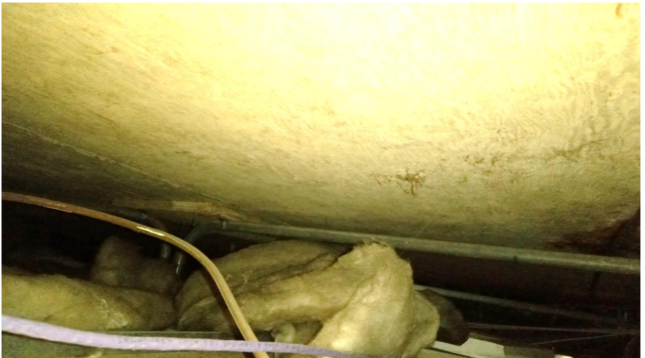
Photograph 10. (Location 1 in the central corridor area), shows the soffit of the roof with restricted space above the ceiling and numerous services / insulation etc.
