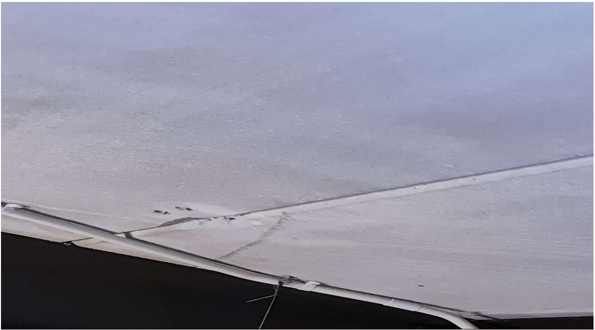
6. Damage to slab edge
