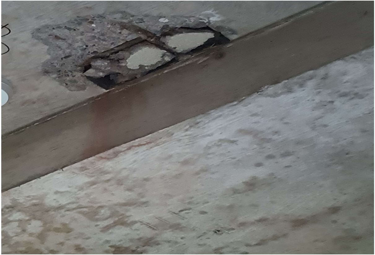
7. Damage adjacent side bearing
