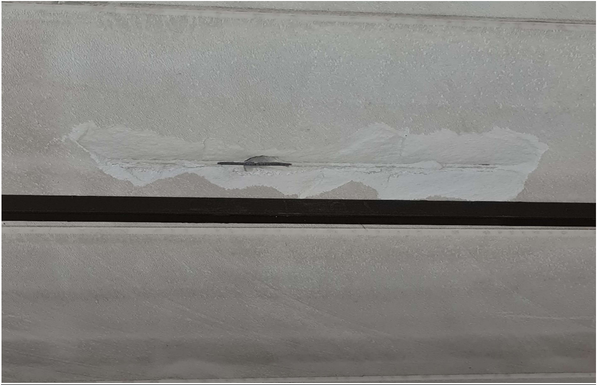
5. Exposed length of the exposed reinforcement
