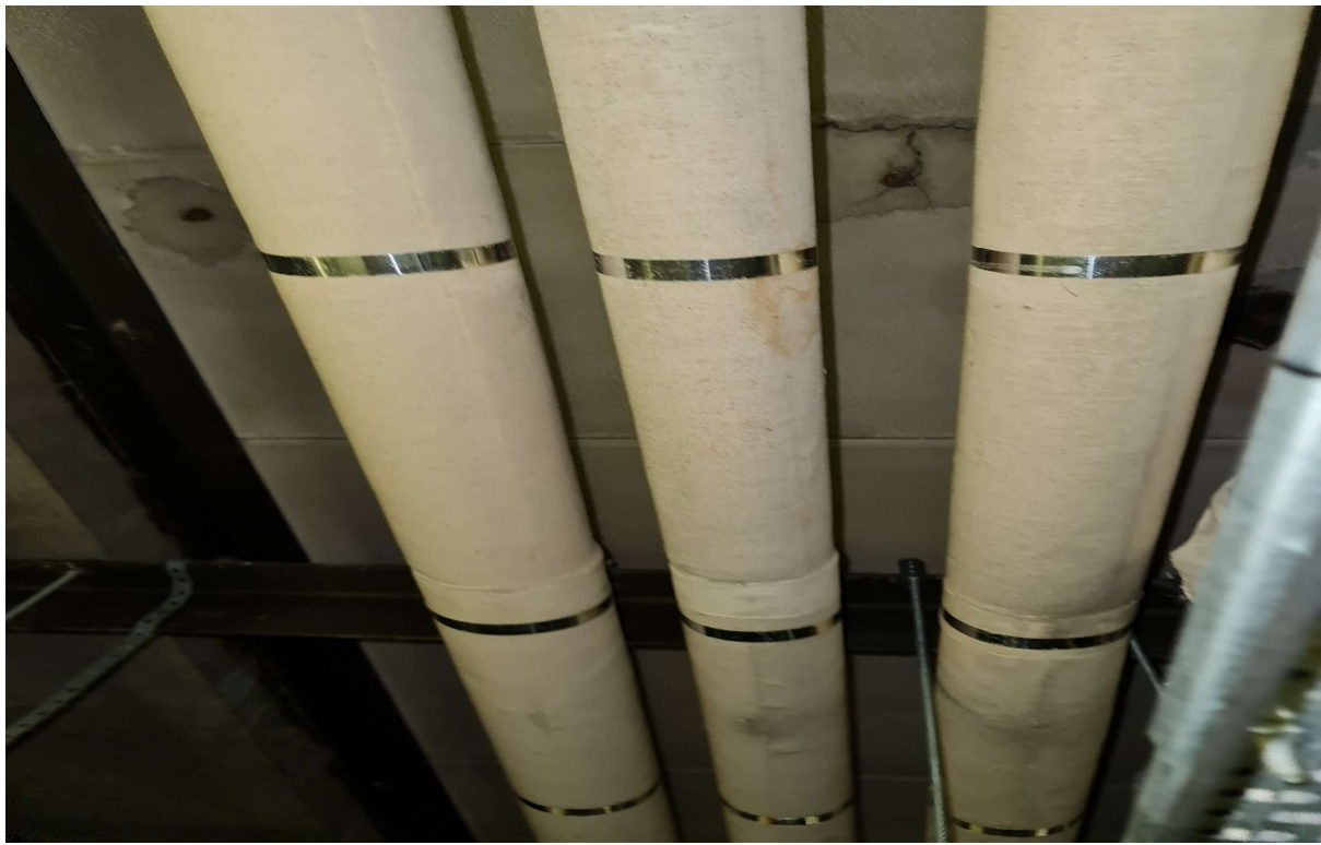
10. Existing patch repairs
