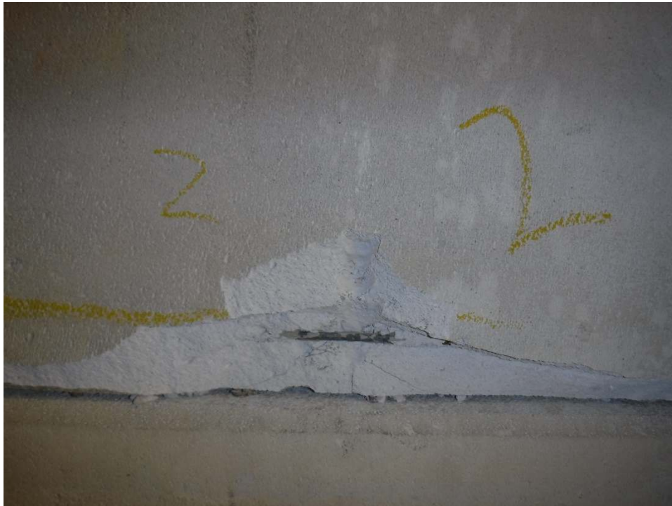
Photograph 008 – Breakout to RAAC planks above plant area
