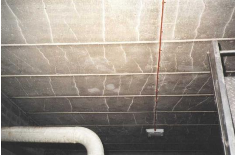
Figure 1 Hairline cracking to soffit of planks
