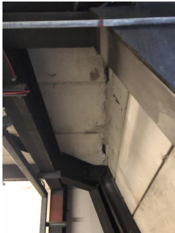
Photo 7 Plant Room 2 - Plank end alterations
