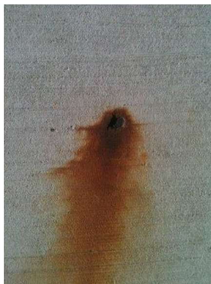
Figure 2 Example of rust staining
