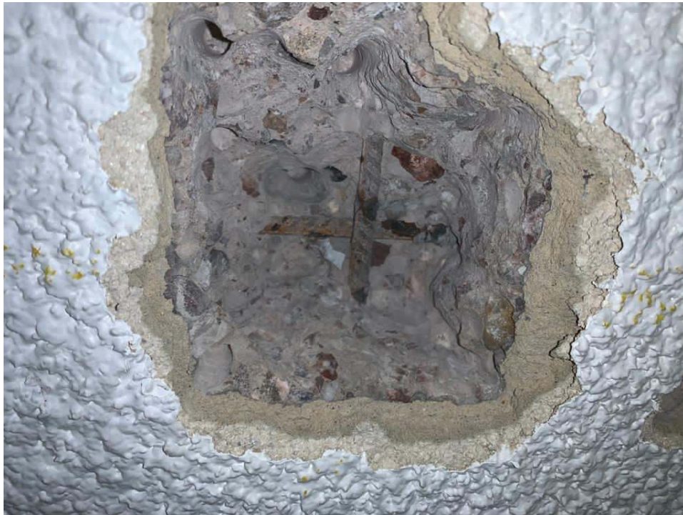
Photograph 004 – Breakout to soffit of hydrotherapy room
