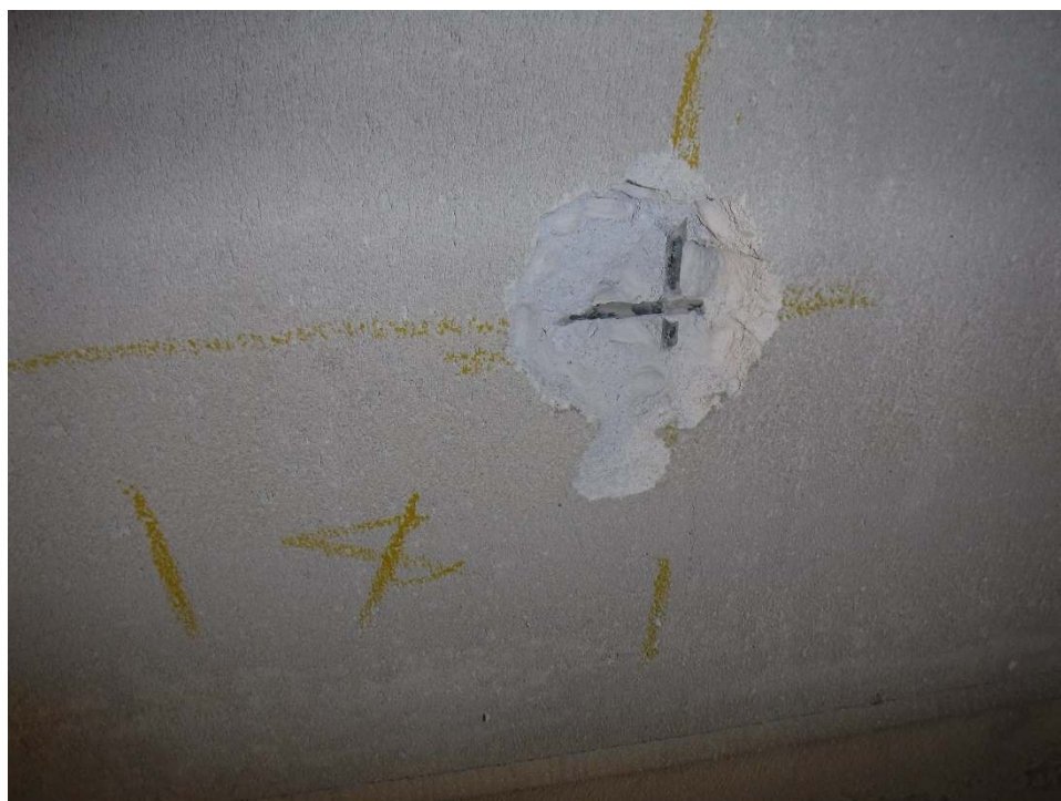
Photograph 007 – Breakout to RAAC planks above plant area
