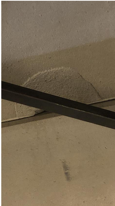
Photo 4 Plant Room 1 Planks - Minor Abrasions
