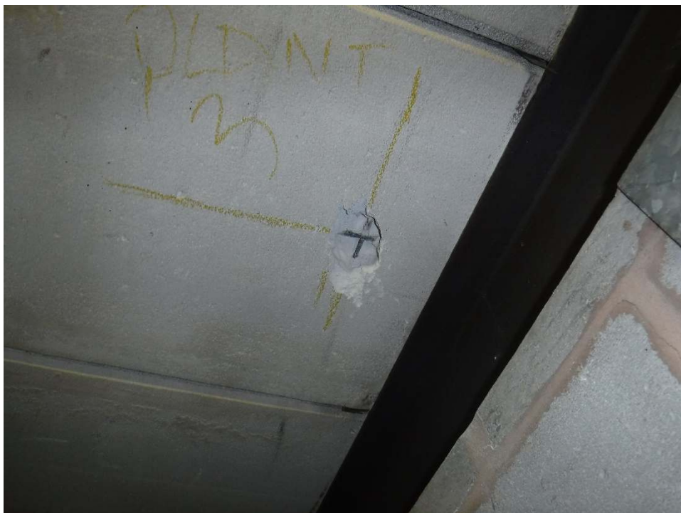
Photograph 009 – Breakout to RAAC planks above plant area
