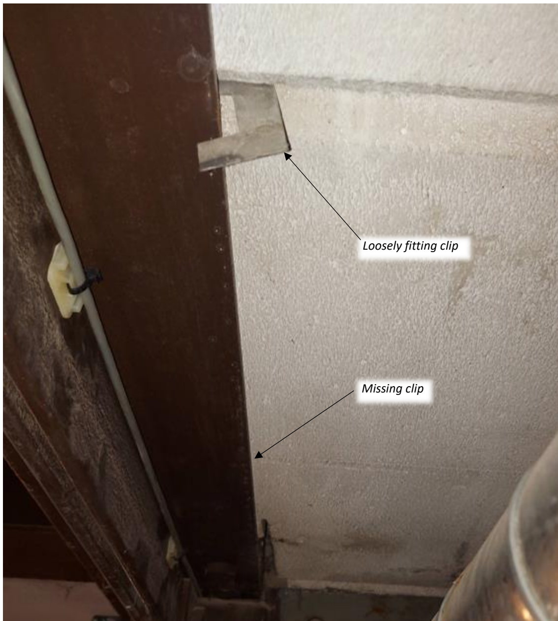
PHOTO 6 – MISSING PLANK CLIPS FOR HOLDING DOWN
