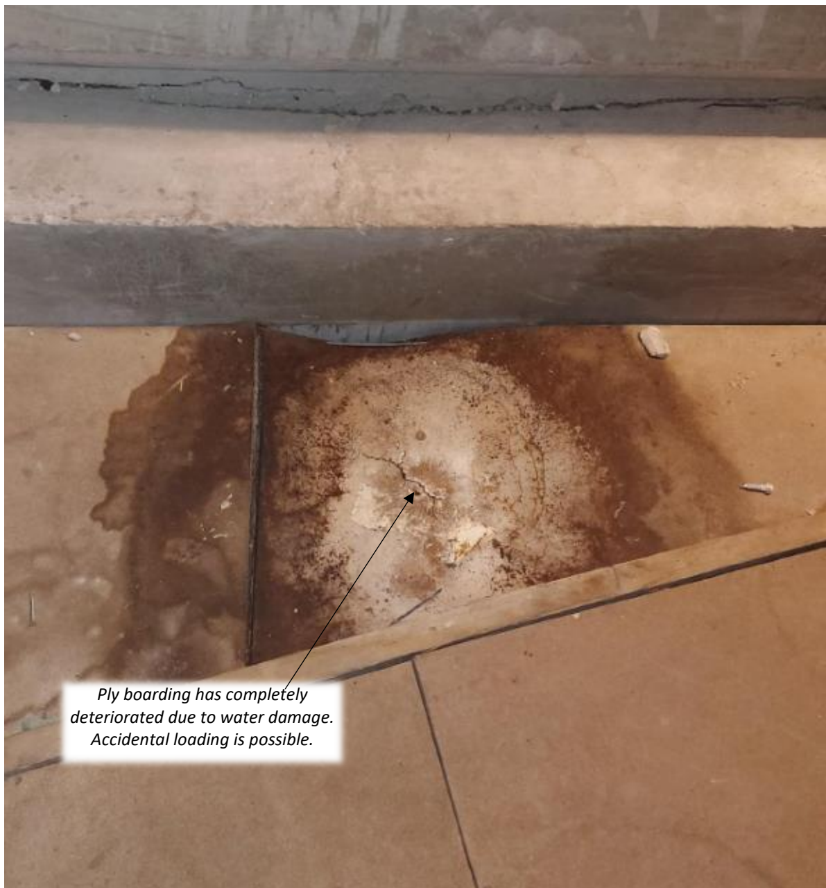
PHOTO 1 – SEVERE WATER DAMAGED PLY BOARDING
