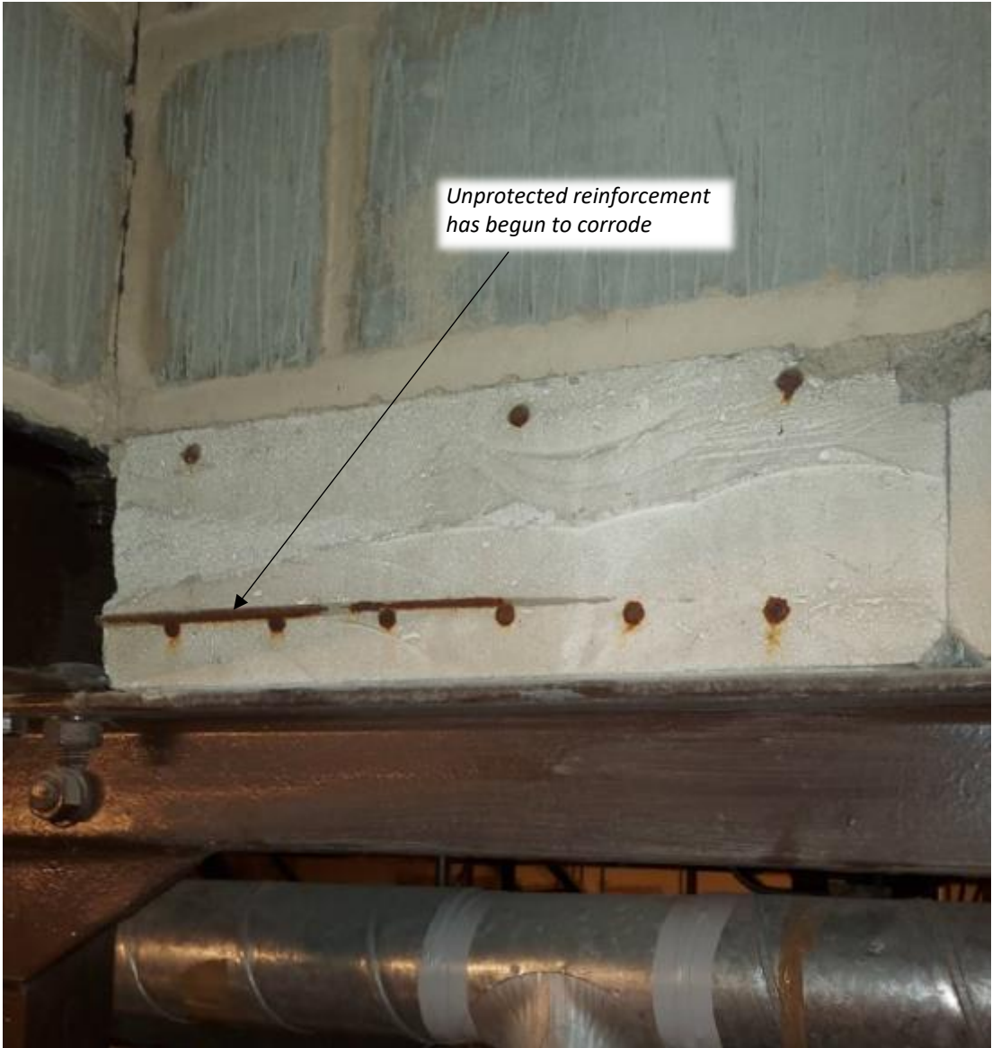
PHOTO 5 – CORROSION OF UNPROTECTED REINFORCEMENT
