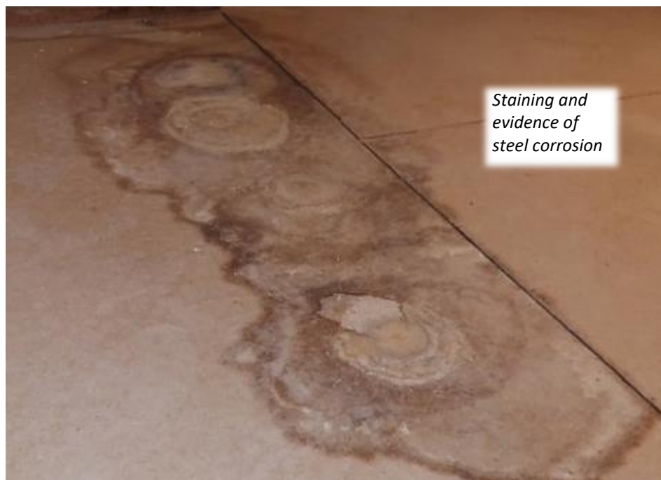
PHOTO 8B – MODERATE WATER DAMAGE BELOW WATER INGRESS LOCATIONS
