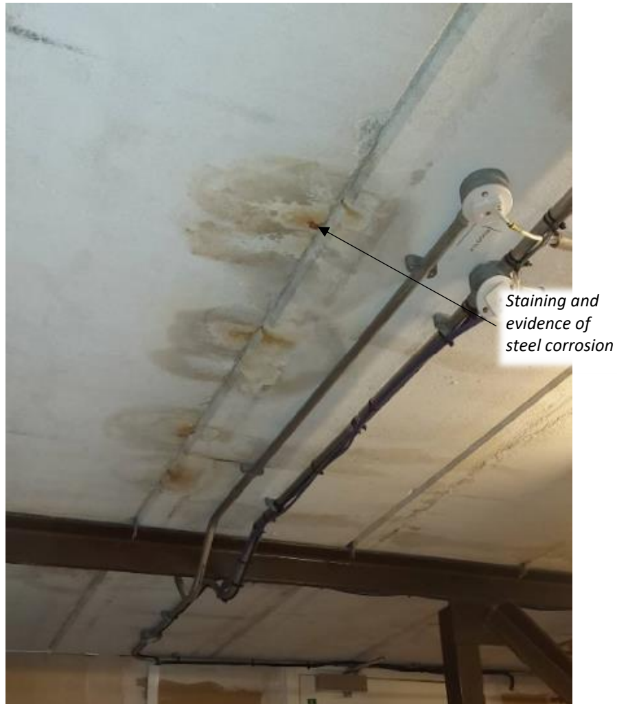
PHOTO 8A – WATER INGRESS AND STAINING OF PLANKS
