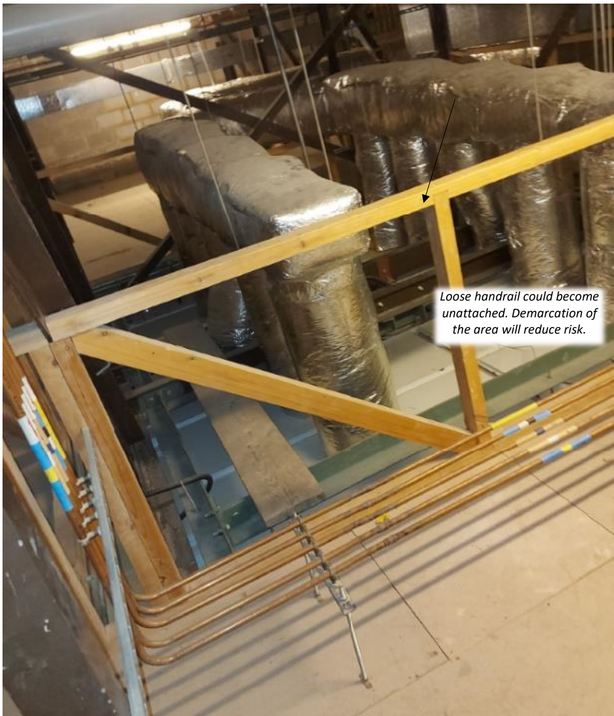
PHOTO 3 – LOOSE HANDRAILS
