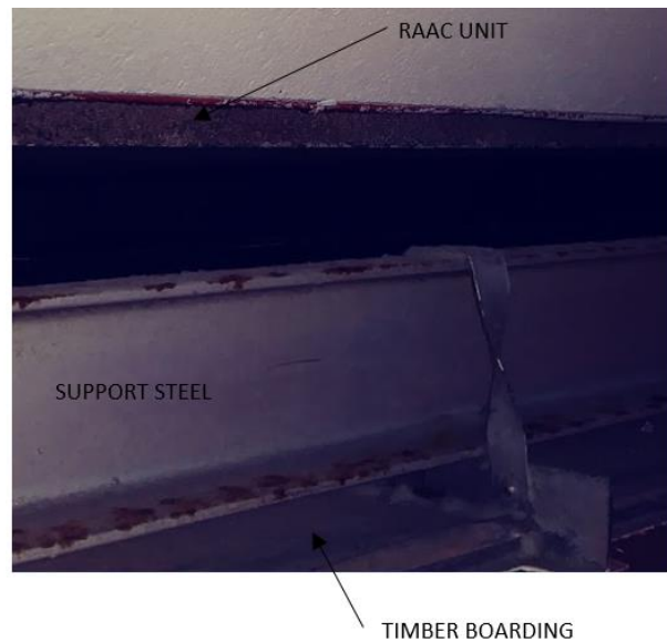
GENERAL ARRANGEMENT OF FLAT ROOF AREAS
