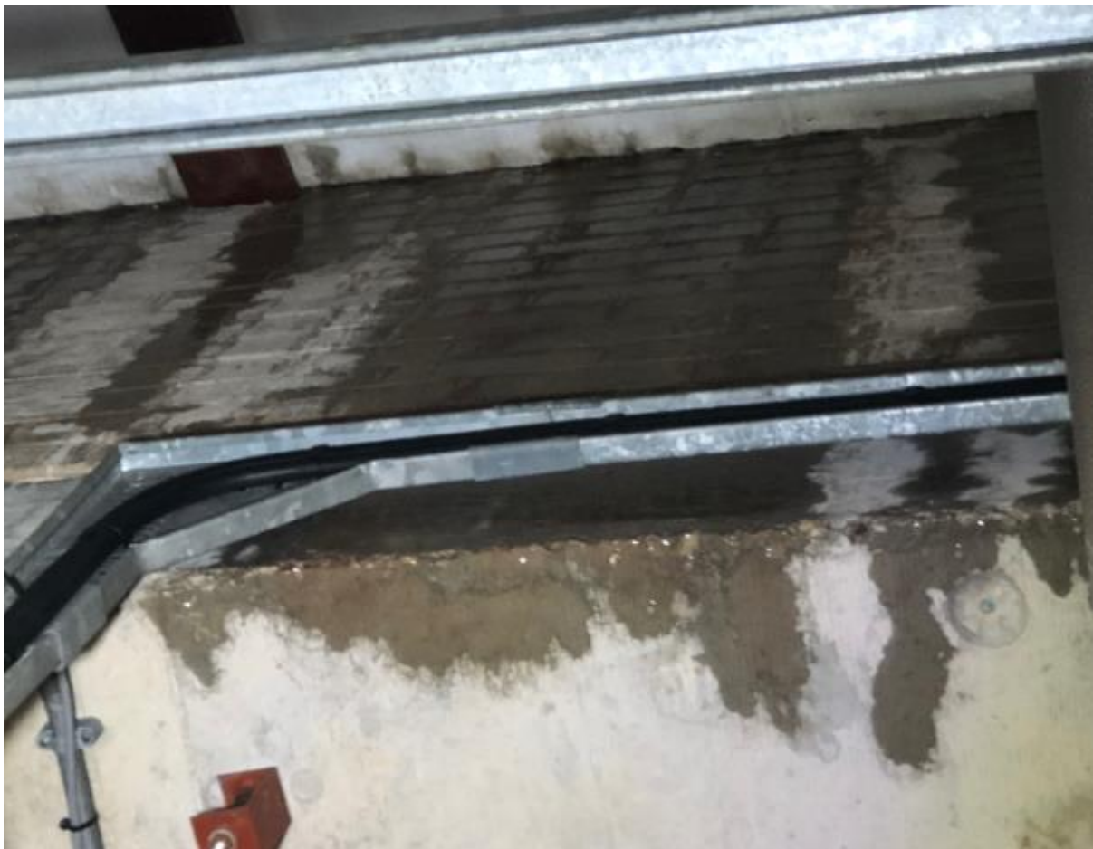
WATER INGRESS DUE TO ROOF LEAKING
