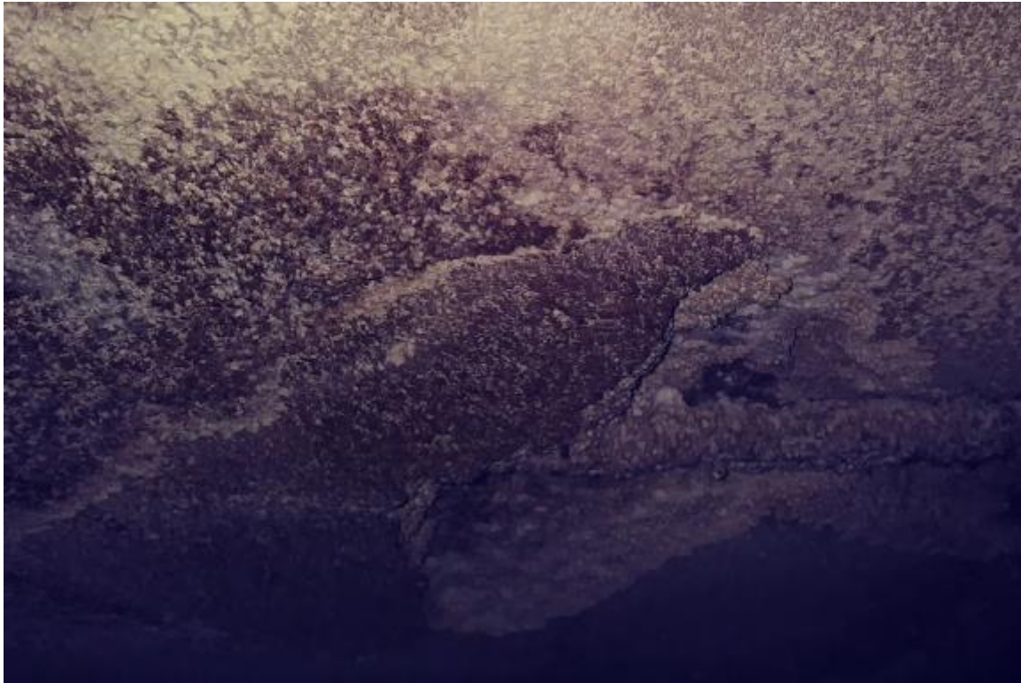
SPALLING OF CONCRETE NEAR ROOF COWL
