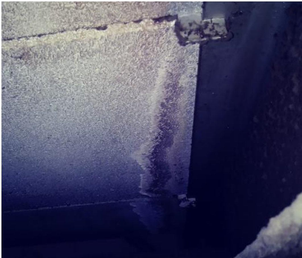
SPALLING CONCRETE AT SUPPORT
