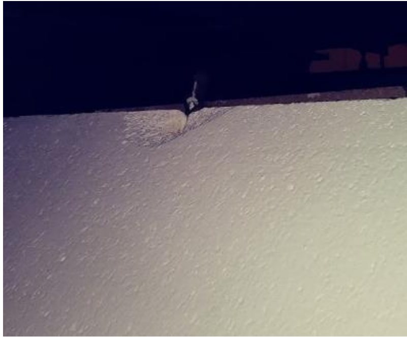
BROKEN CONCRETE AT FIXING LOCATION
