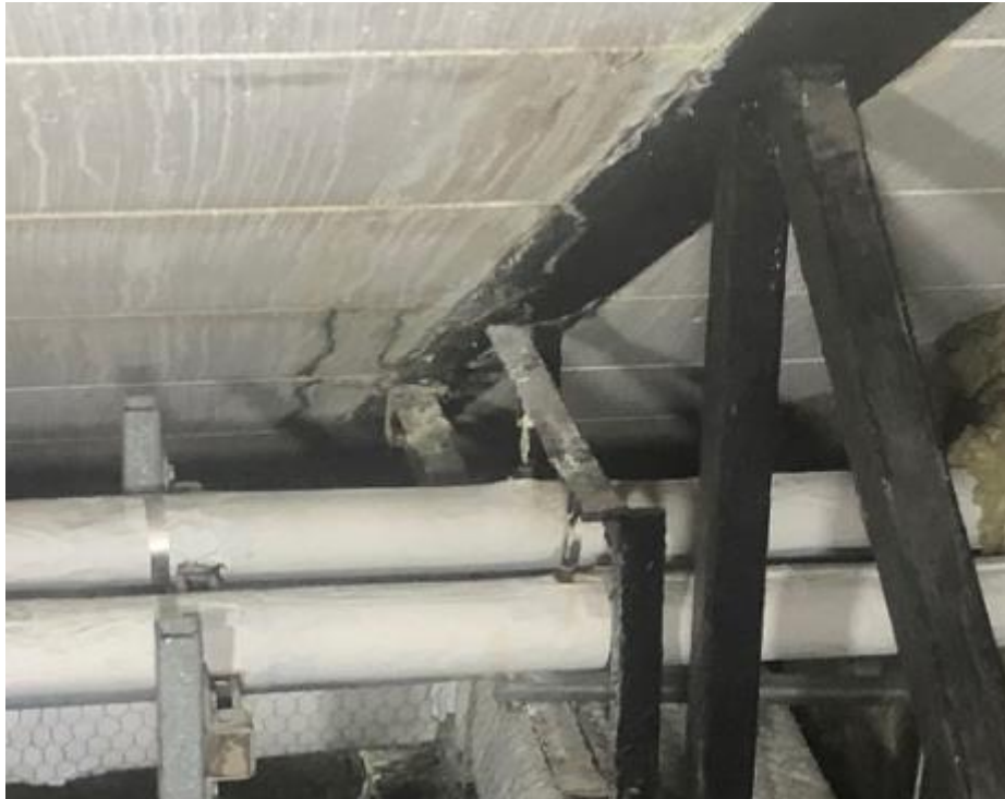
MATERIAL STAINING DUE TO ROOF LEAK
