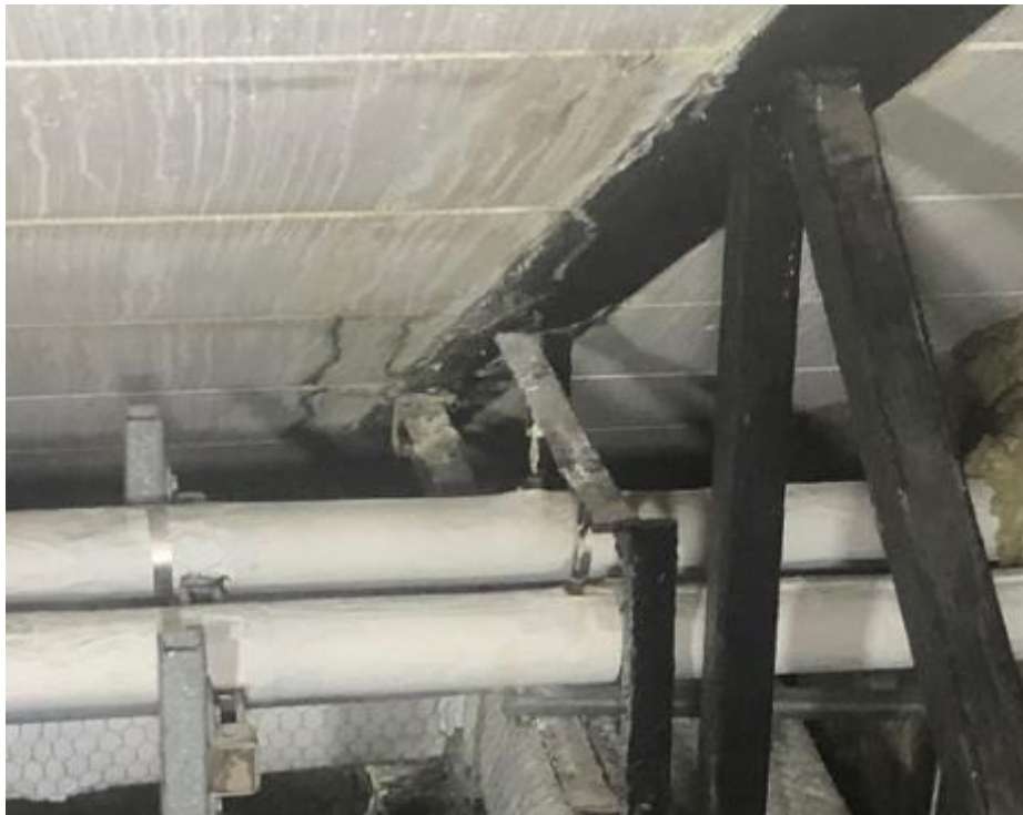
MATERIAL STAINING DUE TO ROOF LEAK
