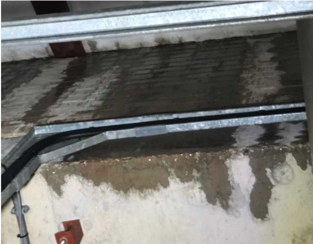
WATER INGRESS DUE TO ROOF LEAKING
