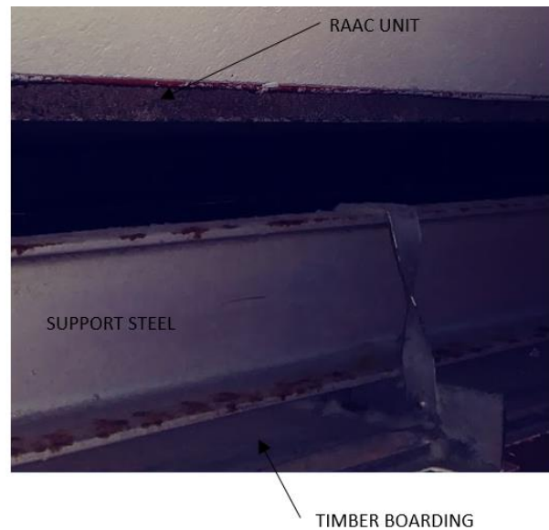
GENERAL ARRANGEMENT OF FLAT ROOF AREAS
