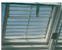
Roof smoke vents (automatic or manual)
